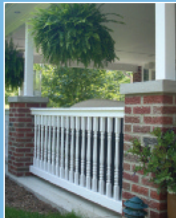
BETWEEN BRICK COLUMNS
