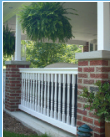
BETWEEN BRICK COLUMNS
